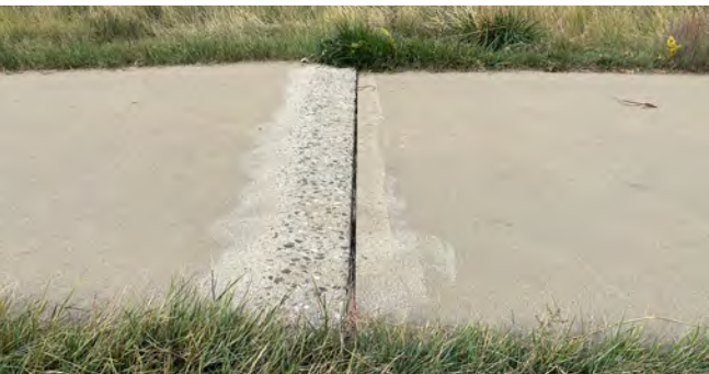
Figure 5 Heaved or buckled sidewalks can be ground down to meet ADA compliance.
