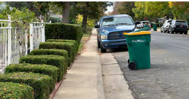
Figure 4 Pre-ADA sidewalks are common throughout the region, and are insufficiently wide for wheelchairs and mobility devices.
