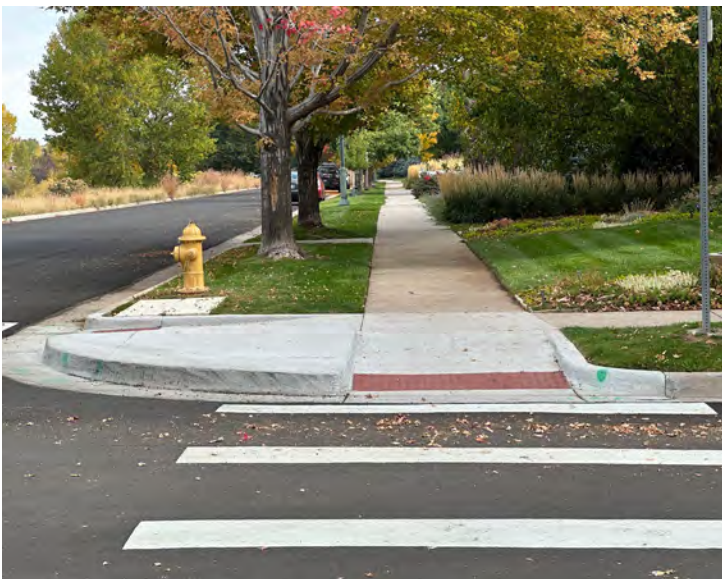
Figure 17 Example of an accessible curb ramp.
