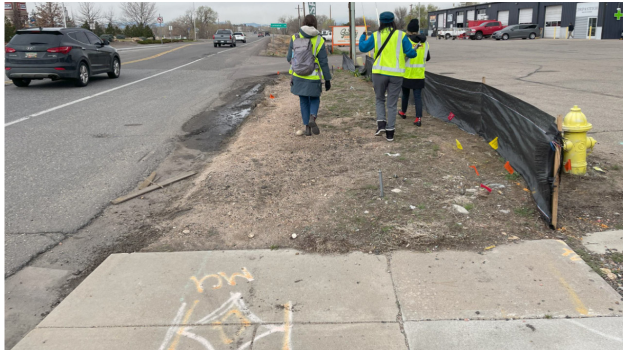
Figure 1. Missing and Deficient Sidewalk Conditions along Bridge Street
