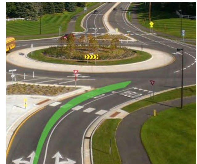
Roundabout with a Mountable Curb
