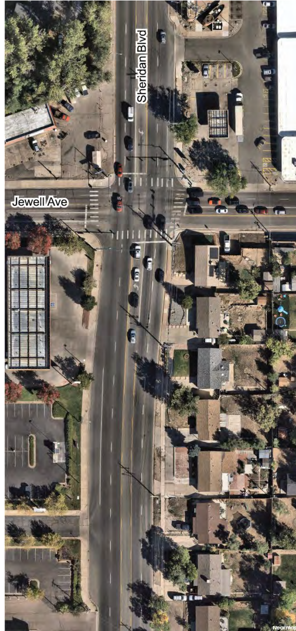
Figure 32. Aerial view of the Sheridan Boulevard and Jewell Avenue intersection.
