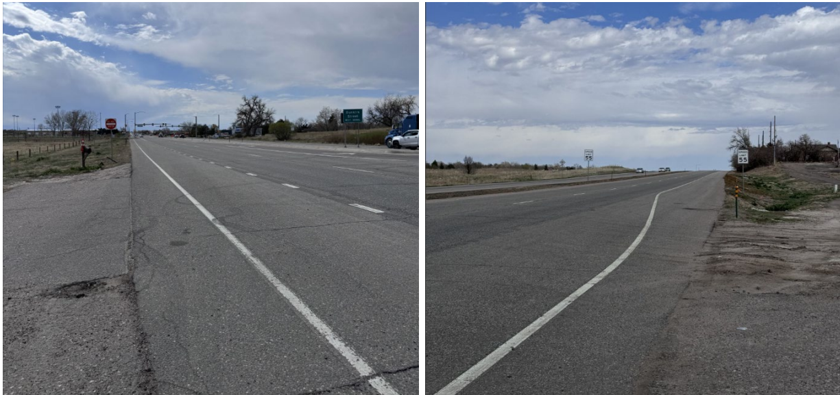
Figure 3-5: Tower Road to E-470 condition photos
