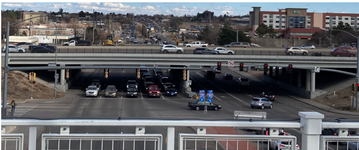
Source: Bespoke Transit Solutions Figure 6-4: I-225 underpass
