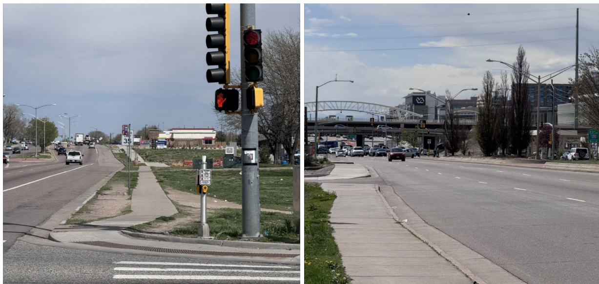
Figure 3-1: I-225 to Chambers Road condition photos
