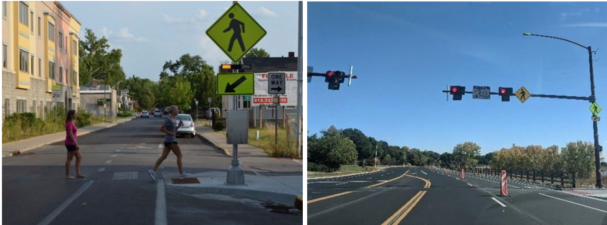
Rectangular rapid flashing beacon, also known as RRFB (left) and pedestrian hybrid beacons, also known as PHB (right)
