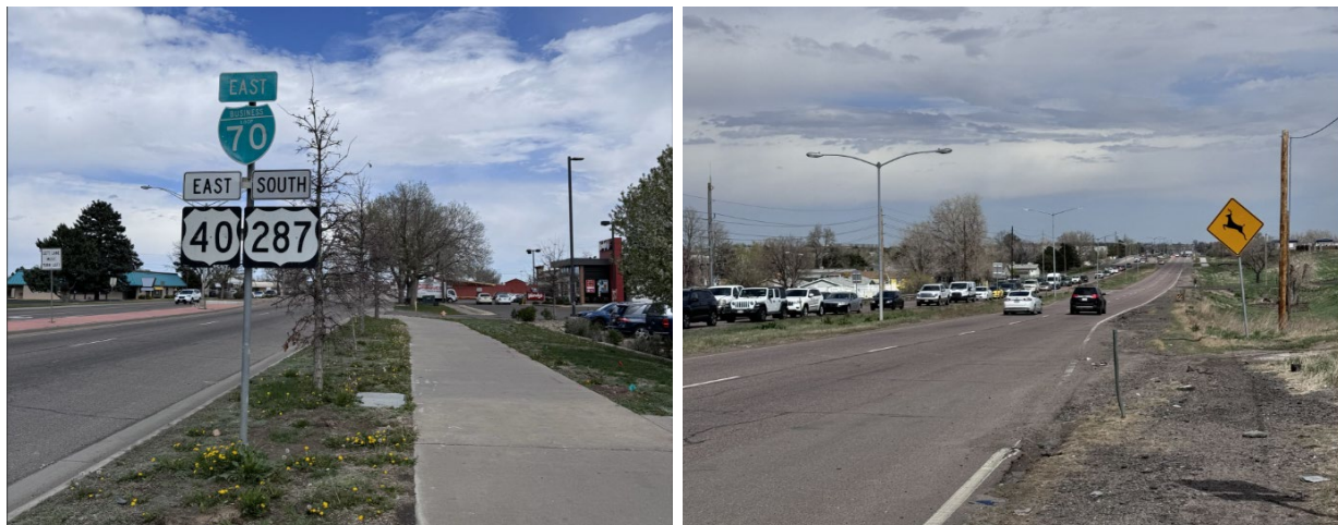
Figure 3-3: Chambers Road to Tower Road condition photos
