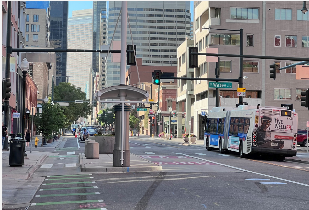
Semi-dedicated lane on 18 th Street in Downtown Denver; Photo Credits: Consultant Team
